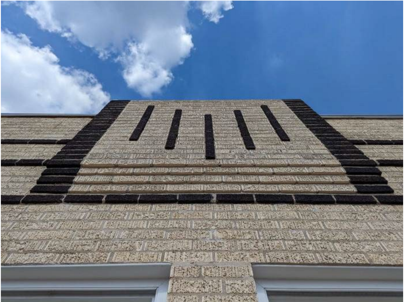
Photo 2: Stepped center bay at West Façade (Front). 17 February, 2023
