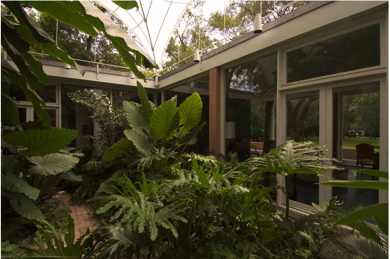
Photo 6: Interior view of the courtyard topped by the canopy roof structure of the Menil House, camera facing southeast. Photo by applicant, 2024.
