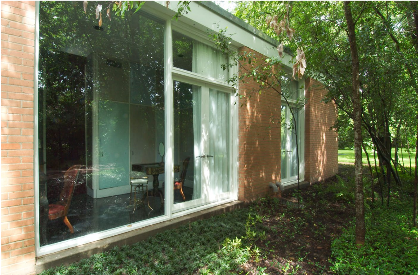
Photo 9: Northeast corner detail of the east side elevation of the Menil House, camera facing northwest. Photo by applicant, 2024.
