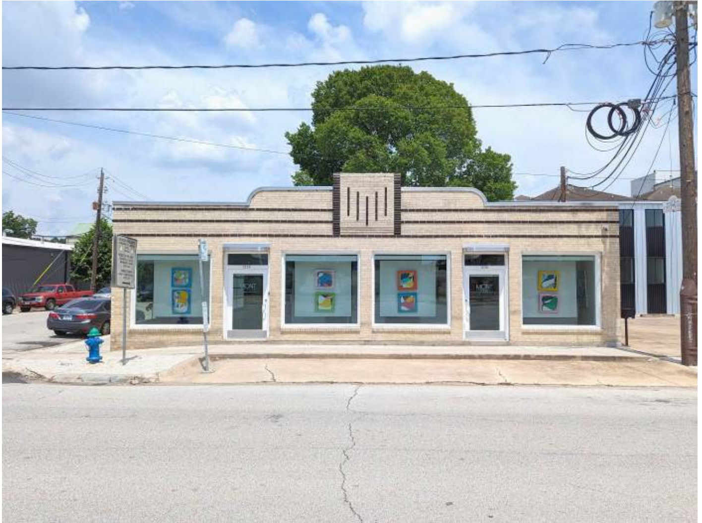
Photo 1: West (Front) Facade from Houston Avenue. 8 June 2023.
