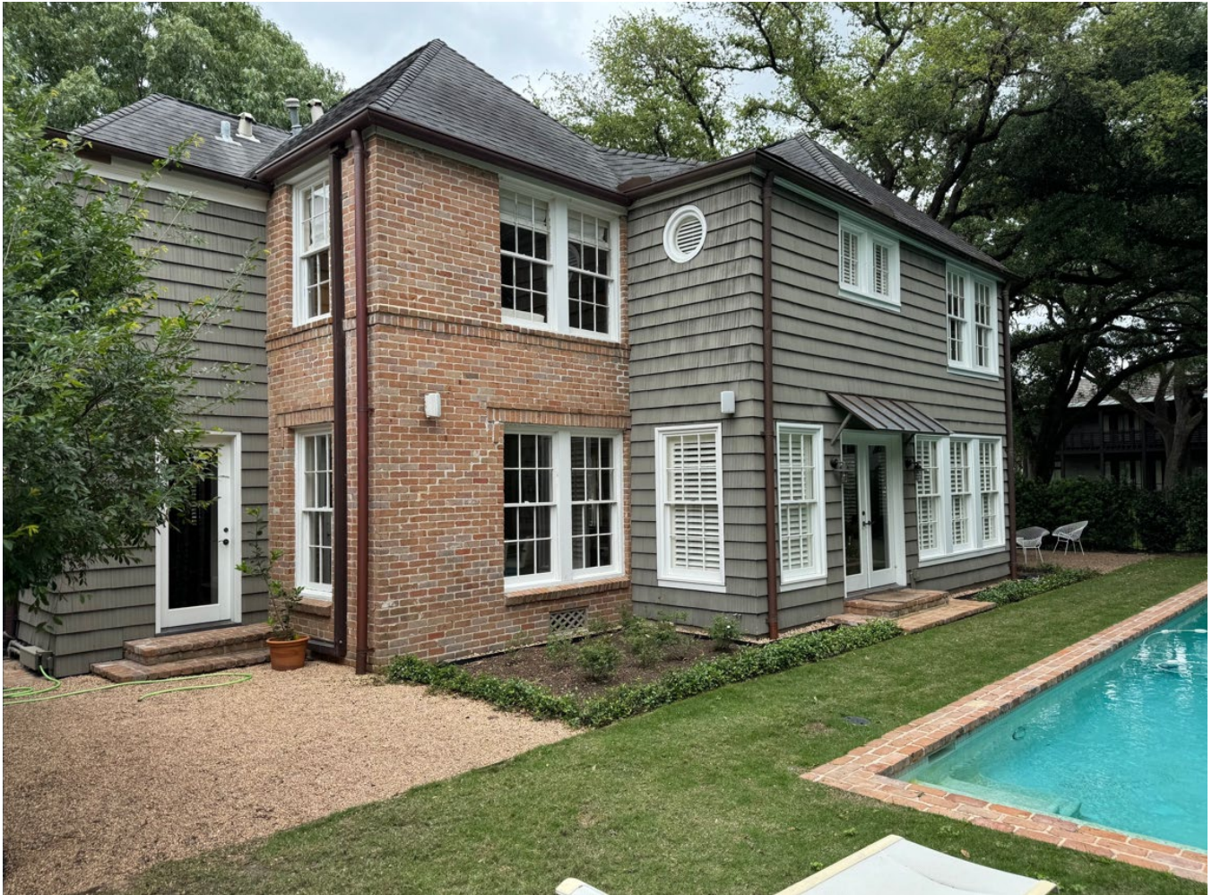
Photo 4: Oblique view of the south (rear) elevation of the Frank A. Watts House, which includes the location of the later wood shingle clad addition. Camera facing northeast. Photo by applicant, 2024.
