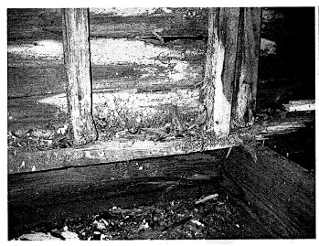
Figure 11: Typical Sill Plate Damage
