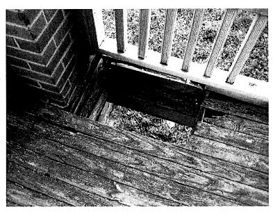
Figure 16: Rotted Porch Deck and Joists
