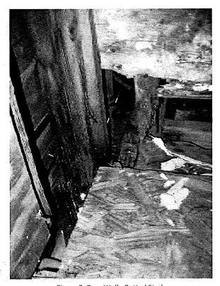
Figure 8: Rear Wall - Rotted Studs
