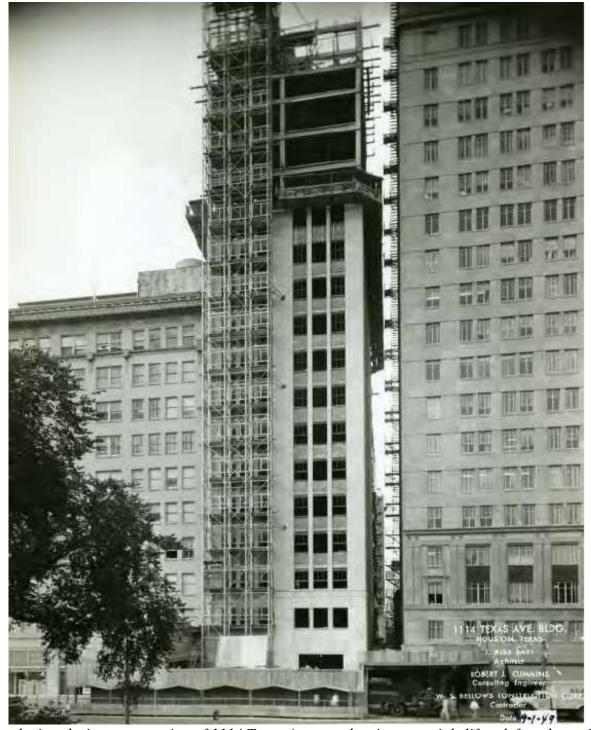
North view during construction of 1114 Texas Avenue, showing materials lift at left and exterior suspended platform at right.
