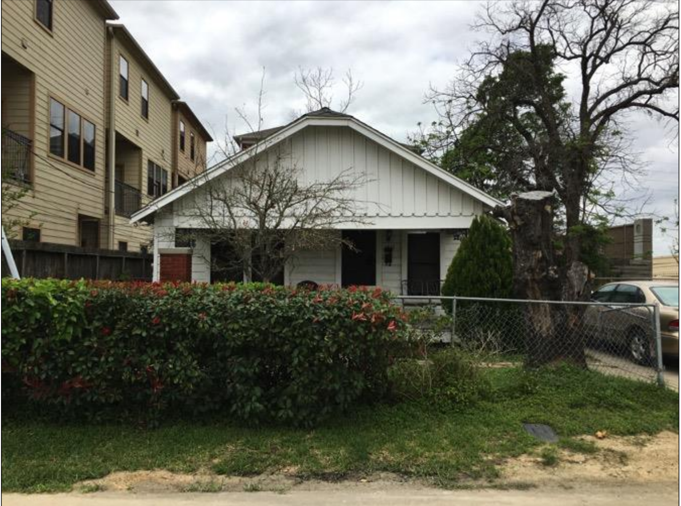
East façade facing west on Bass St. Photos by Cory Johnson, City of Houston.
