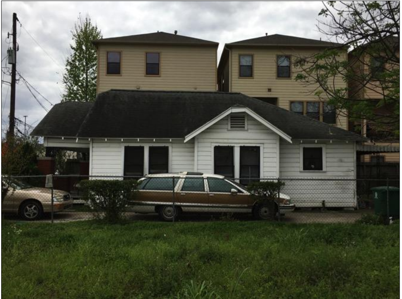
North façade facing south on Katy Freeway Service Road. Photos by Cory Johnson, City of Houston.
