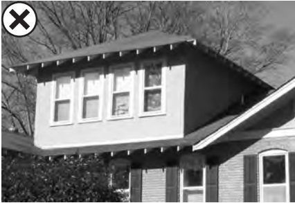
This dormer overwhelms the house and is inappropriate.
