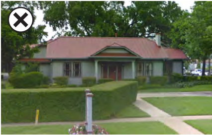
The red metal roof on this house is more appropriate for a commercial building, not a residential one.
