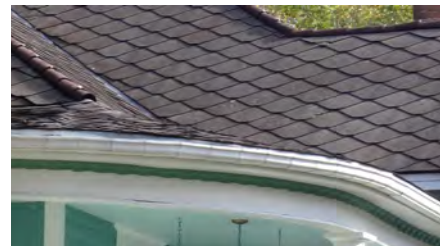
Asbestos-cement shingles have an estimated 50–70 year service life.
