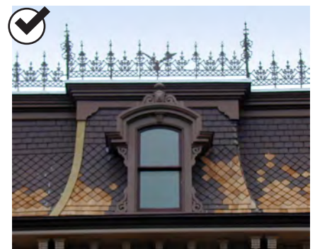
Patch and replace damaged areas of the existing roof.
