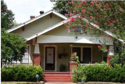
A front gabled roof
