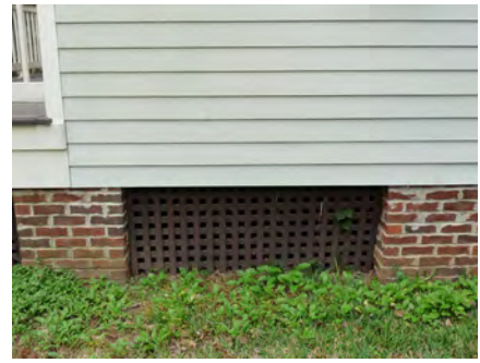
A foundation with masonry piers
