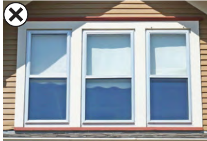
Unfinished metal windows such as these alter the character of window openings, and should not be used in highly visible locations.
