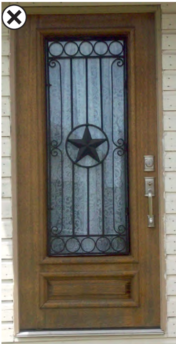
This replacement door with ornate, faux leaded glass would be inappropriate on many historic buildings.
