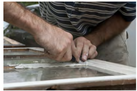
Replacing glazing putty © iStockPhoto.com/Elaine Odell
