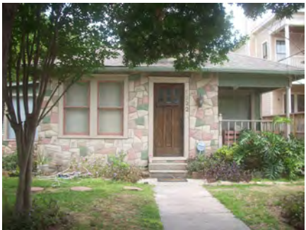
Faux-stone, panelized wall cladding (not appropriate for the Houston Heights Historic Districts)
