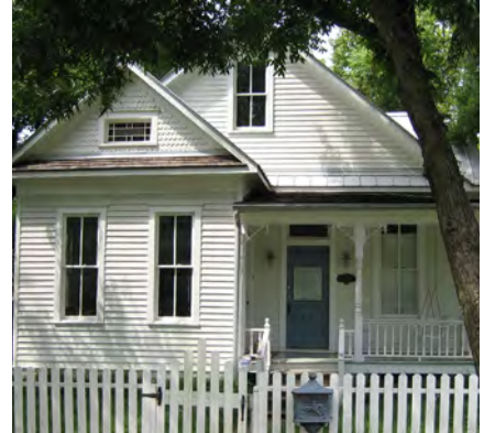
A house with intact historic windows.
