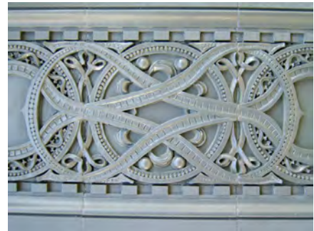
Historically, metals were used for a variety of applications, including columns, roofs, balcony railings, and other decorative features.
