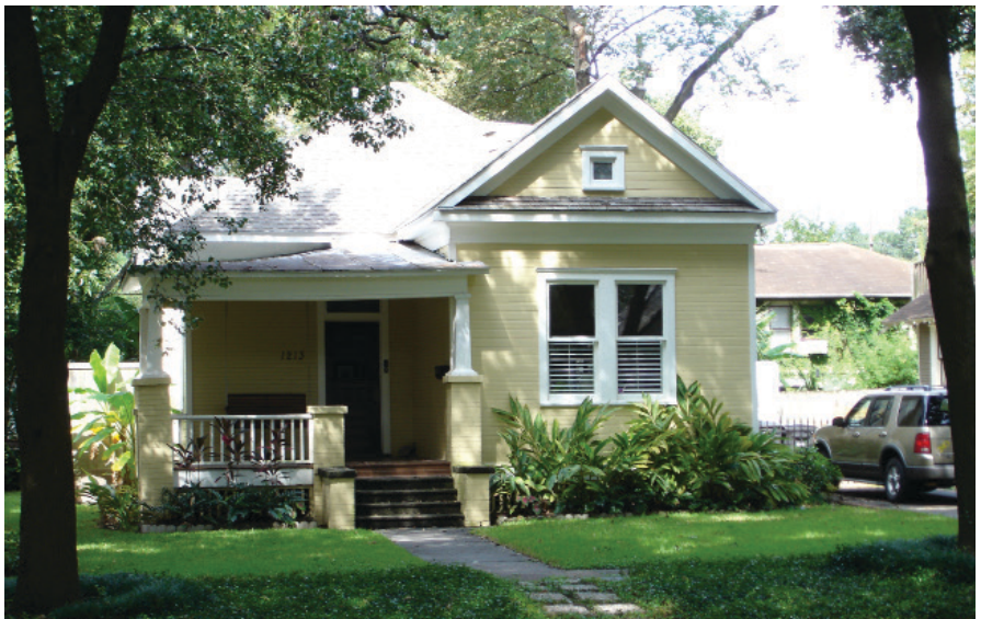
This house at 1213 Harvard Street incorporates a Queen Anne roof form and front door with a Craftsman front porch and paired windows.
