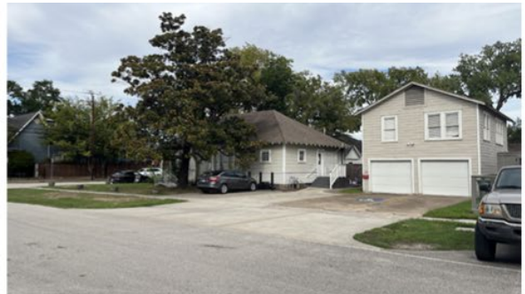
Photo 03 540 Cortlandt West/ South Elevation
