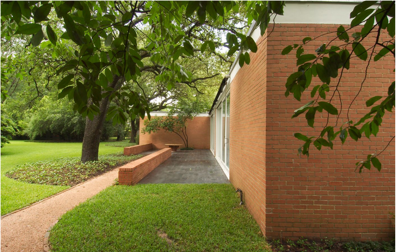
Photo 7: Rear entrance on the southeast corner of the Menil House, camera facing west. Photo by applicant, 2024.
