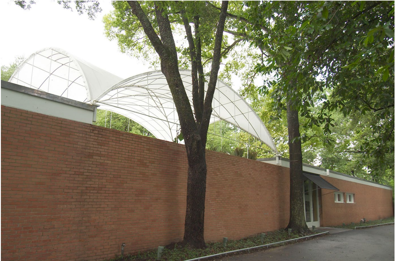
Photo 5: Oblique detail view of the north elevation and courtyard canopy roof structure of the Menil House, camera facing southwest. Photo by applicant, 2024.
