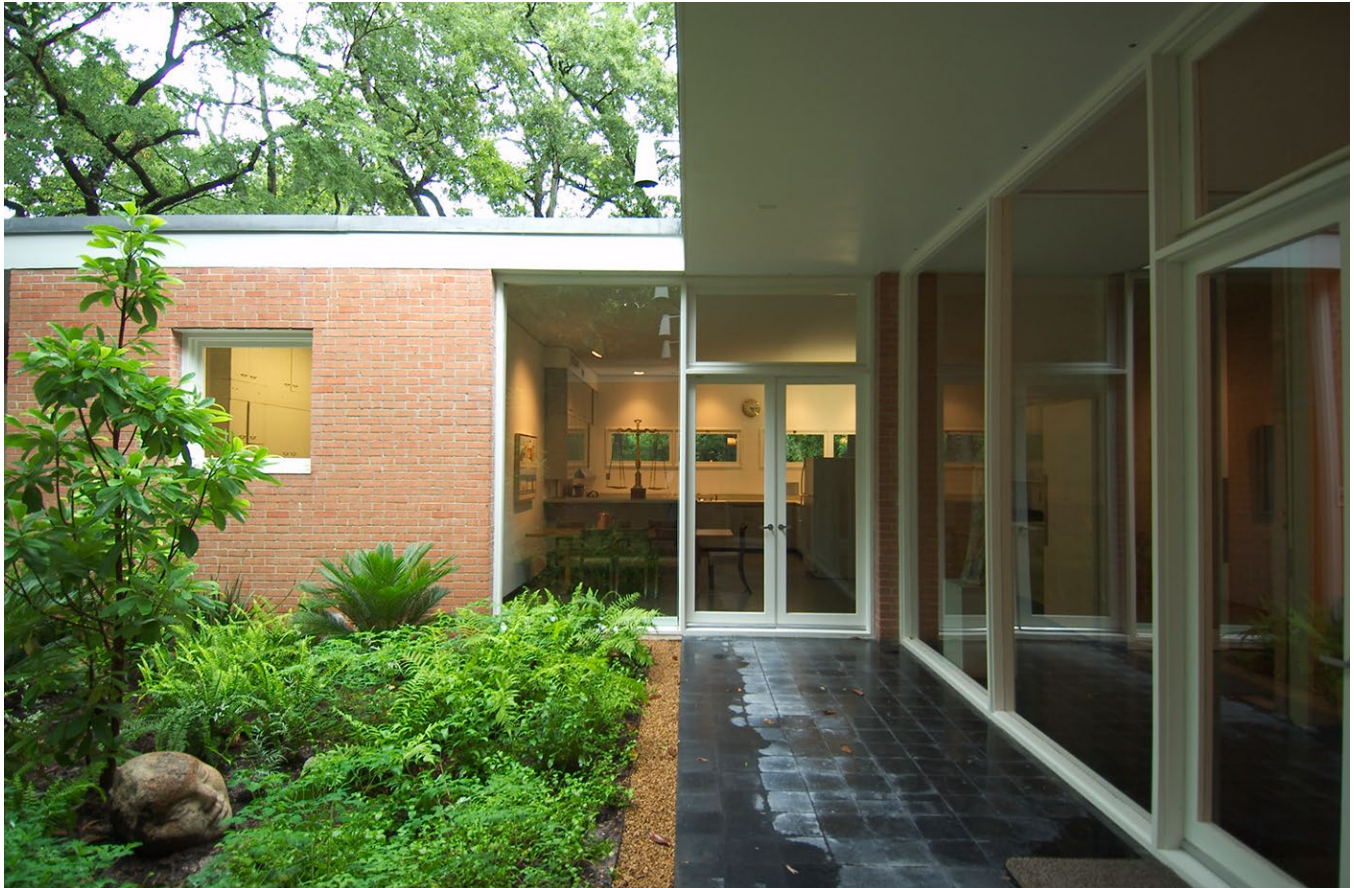
Photo 14: Detail view of the south elevation rear entrance inset on the southwest corner from the rear driveway of the Menil House, camera facing north. Photo by applicant, 2024.
