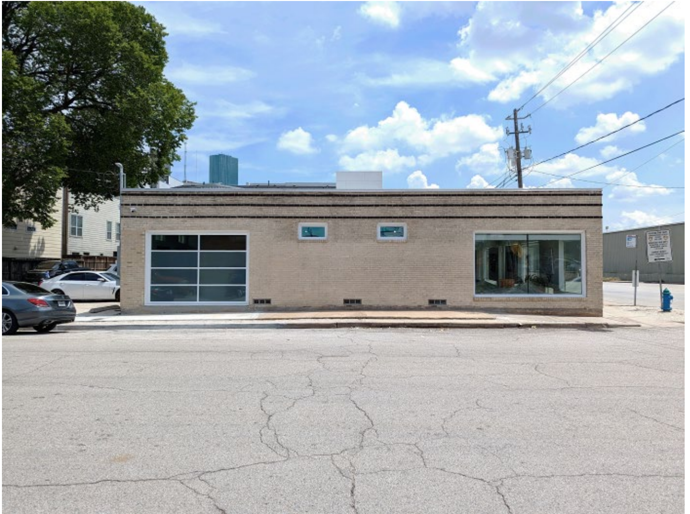
Photo 4: North (Side) Façade facing Dart Street. 8 June 2023
