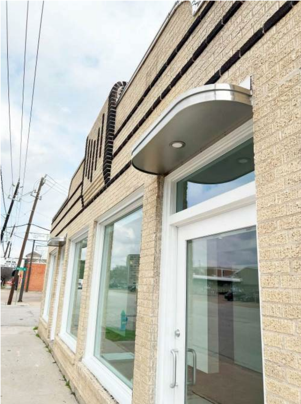
Photo 3: Curved Metal Canopies and Entries at West Façade (Front). 17 February, 2023
