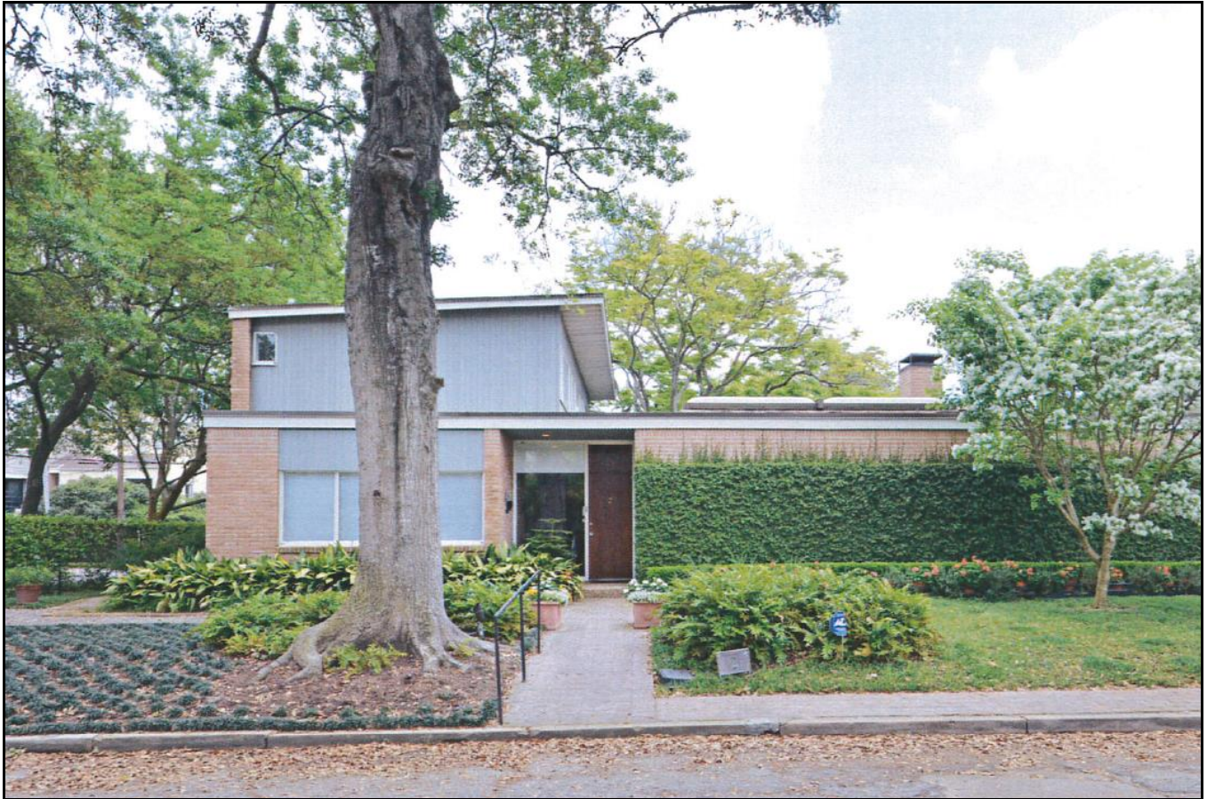
Residence for Mr. & Mrs. S.I. Morris. Front (west) façade looking east from Waverly. 2 Waverly Court, Houston, Harris County Texas 77005. March 31, 2015.
