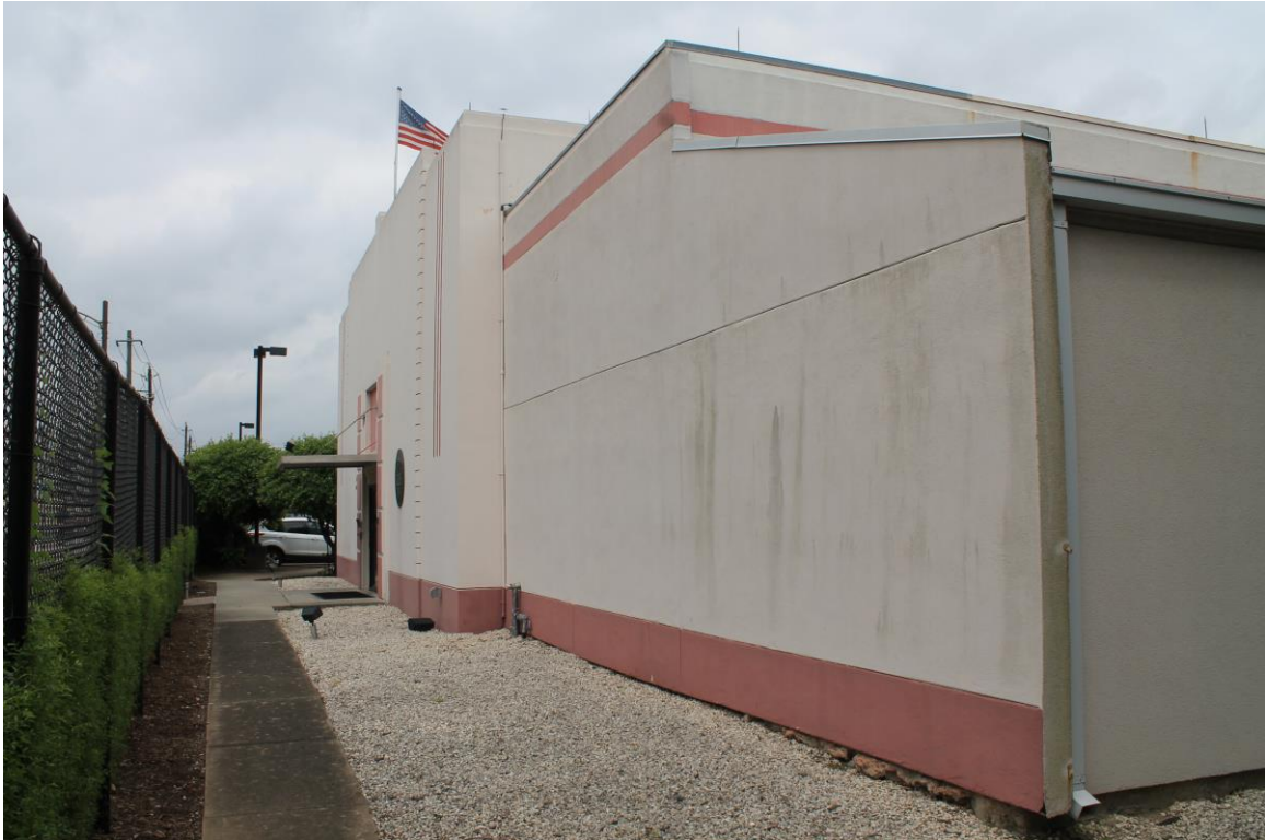
Photo of existing east addition Staff photo, April 3 rd 2015
