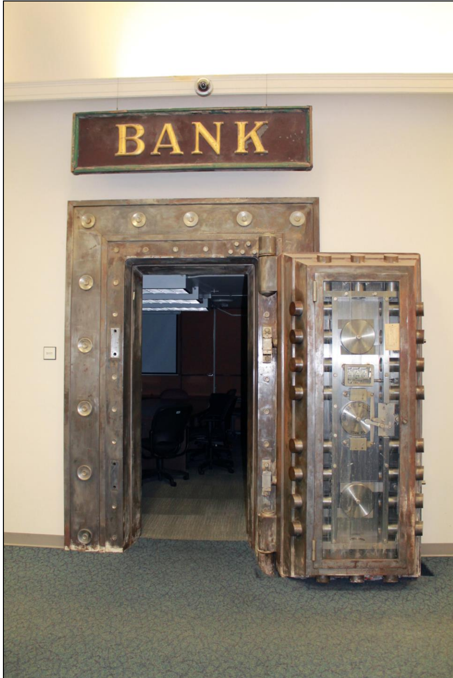
Photo of interior bank vault door Staff photo, April 3 rd 2015
