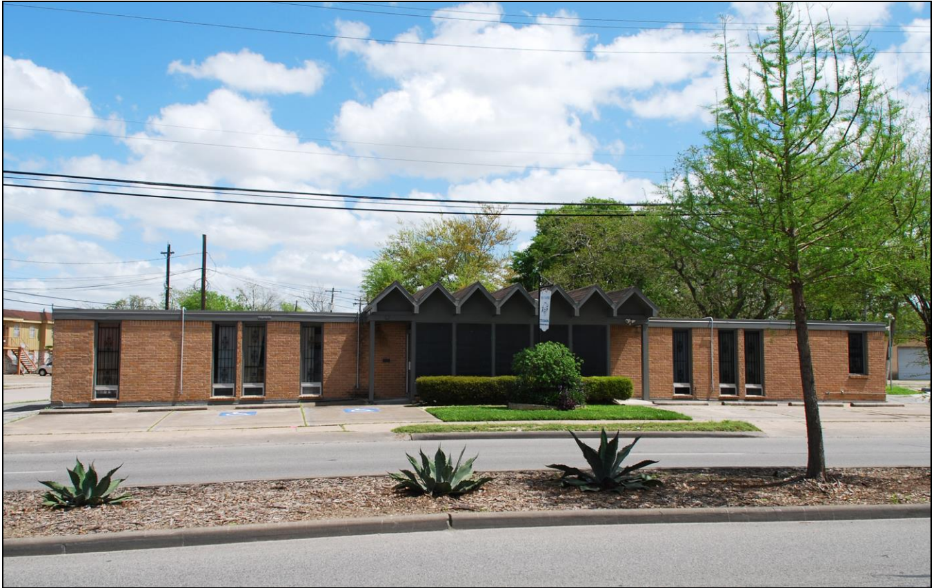
The Cullen Clinic, later known as Poindexter Dental, Inc. View: Looking east across Cullen Boulevard toward front facade Photos by David Bush, Preservation Houston Date: March 29, 2015
