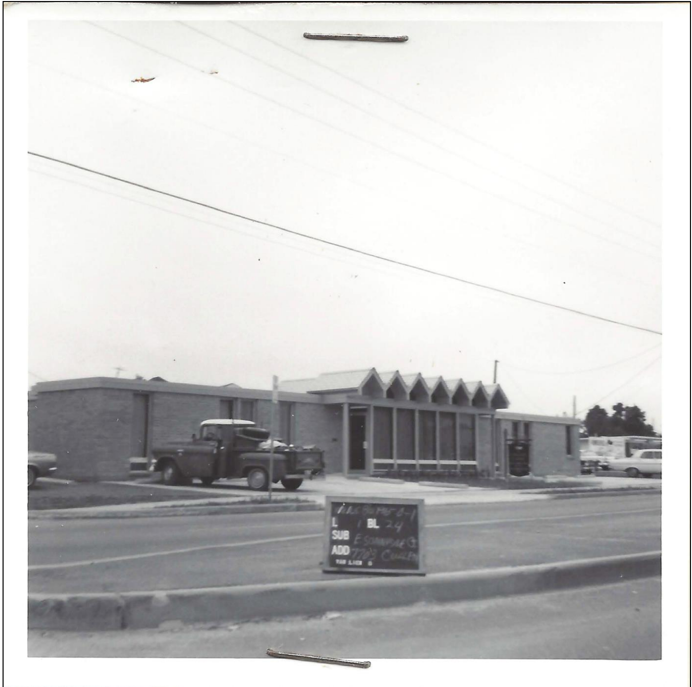
The Cullen Clinic, 7703 Cullen Boulevard, Houston, Texas November 12, 1965 by Harris County Building Assessment Source: Harris County Archives
