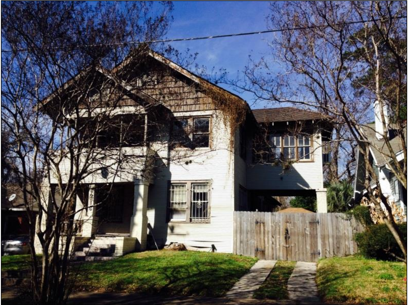
Condition prior to purchase and restoration.
