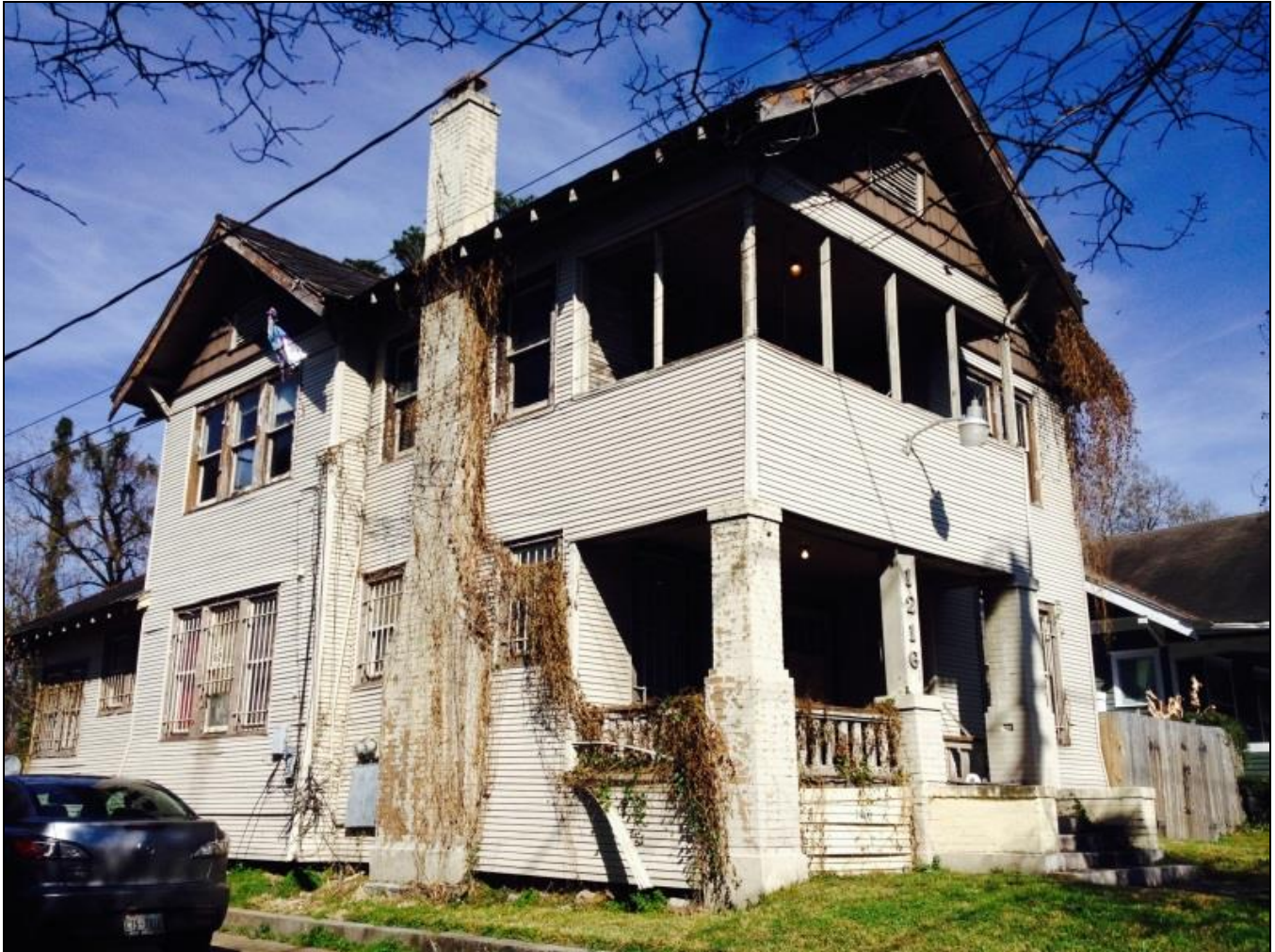
Condition prior to purchase and restoration.
