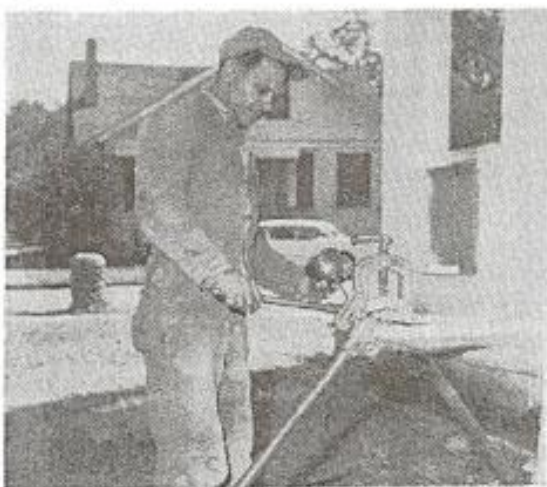
The professional plumbers contributed their work. Shown is Joe Hernandez.
